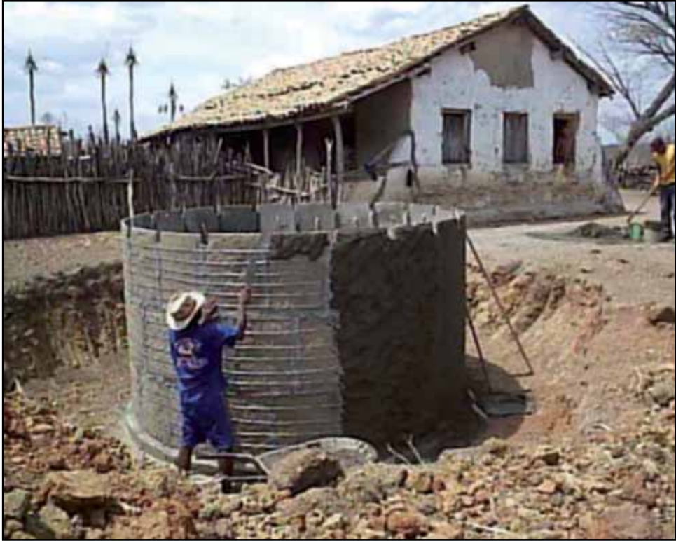
Photo 16 – Aspects of External Plaster of a Rain Cistern
