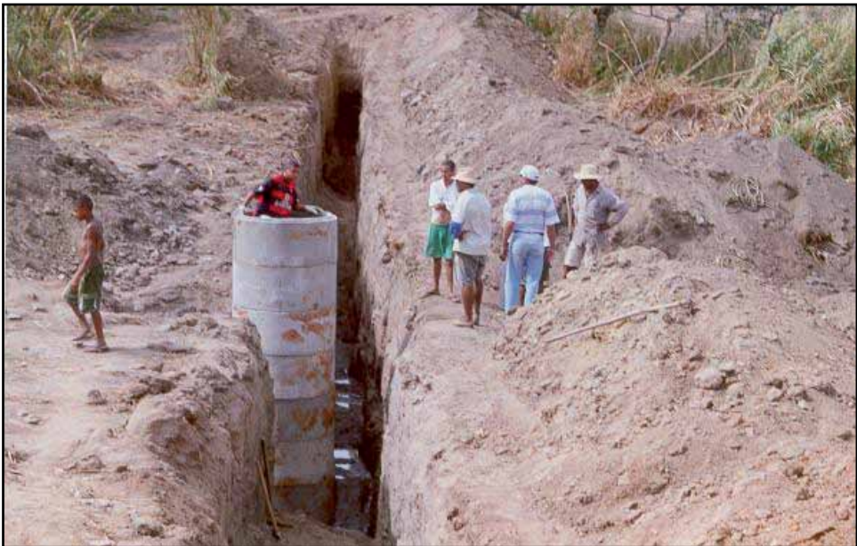
Photo 6 - Aspect of an Underground Dam under Construction
