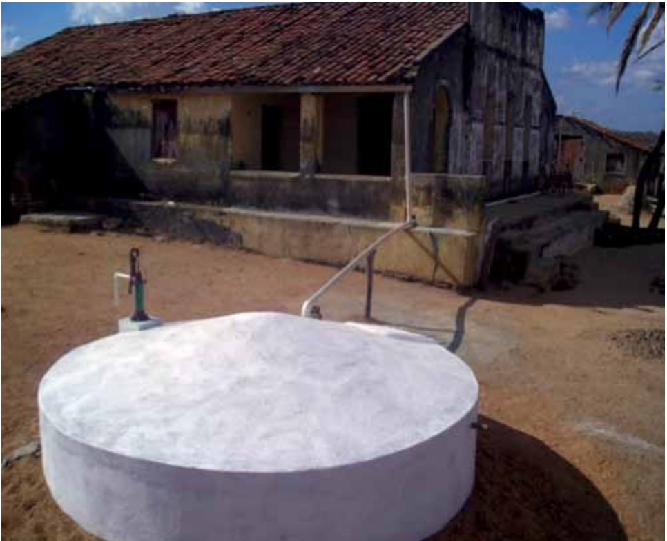
Photo 17 - Rain Cistern Constructed by PRODHAM
