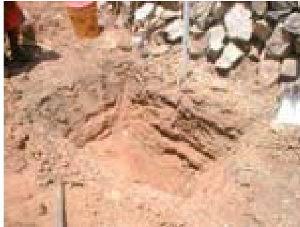
Photo 3.08 – Trench for ruler installation in successive dam
