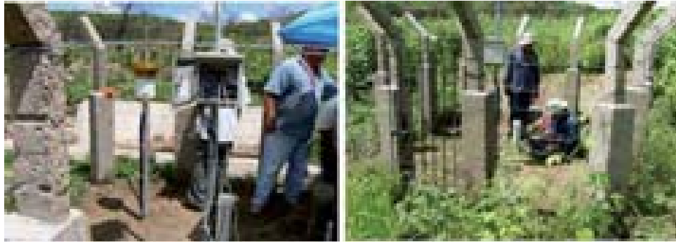
Photo 2.06 – DCP installation in flume 02, data collection and evaluation of equipment calibration.
