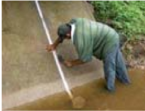
Photo 2.07 – Installation of limnimetric ruler in flume 01
