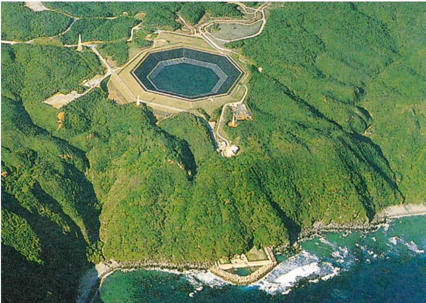
Fig. 1—Bird's-Eye View of Pilot Seawater Pumped-storage Power Plant, Okinawa Pref. in Japan. The octagonal shape shows the upper dam. The sea is the lower reservoir. The outlet of the tailrace is surrounded by tetrapods for protection from waves.
